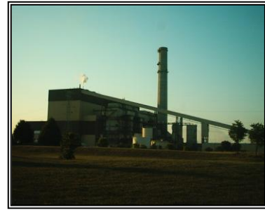
Pleasant Prairie Power Plant, Unit 1-2 Addition
